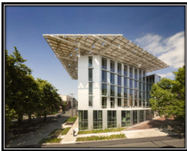
Fig. 3. The Bullitt Center, Washington, USA
