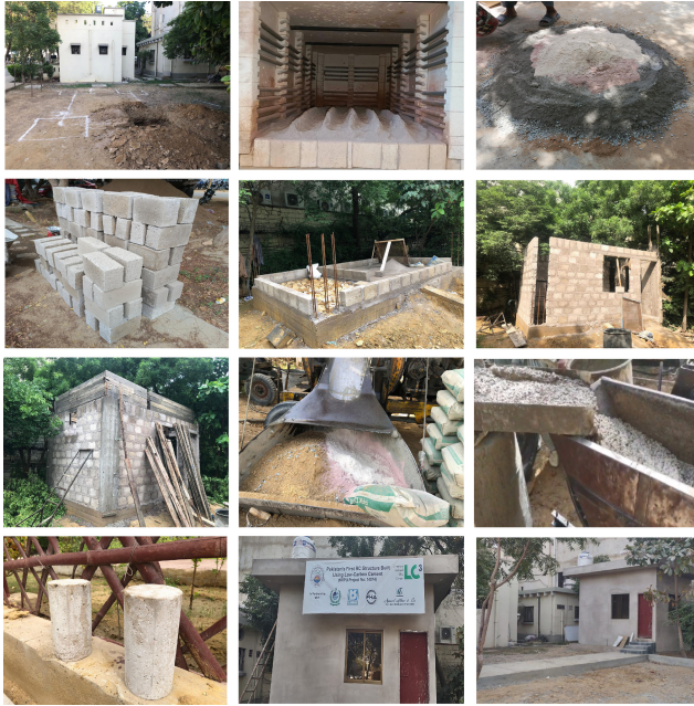
Fig. 3. The entire construction process is depicted sequentially
